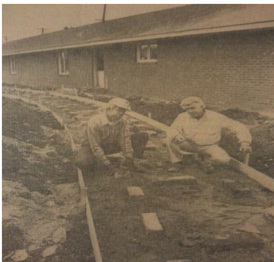
St. Mary's building construction
